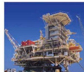
Offshore- FPSO, Drill ship
